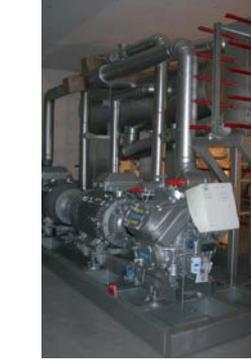
4 units of heat source HP with a capacity of 1,000 kW
