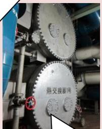
The heat exchanger is made of titanium and a strainer filtrates untreated water in conduit.
