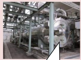
The heat exchanger is made of stainless steel and a strainer filtrates untreated water in conduit.
