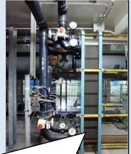
Heat exchanger is a general plate type that does not incorporate any new technological elements of heat exchanger systems.
