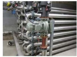
Double pipe sewage water heat exchangers and heat pumps are installed in the equipment room of the multiple-family dwelling. The pipes for heat exchangers have the same diameter of water supply pipes. After heat exchange, garbage flows with sewage.
