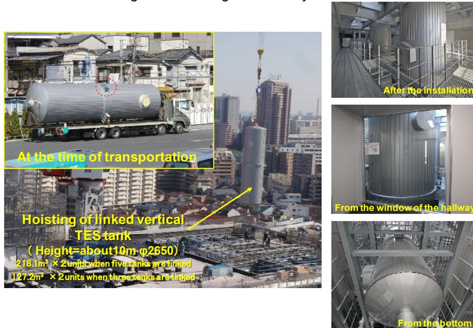
Figure 7: Linked vertical TES tanks
