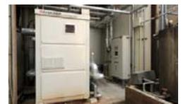
↑ Heat recovery heat pump (water heat source Eco Cute)
