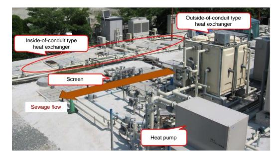
Tests were conducted at Chishima Sewage Treatment Plant in Taisho-ku, Osaka-shi to measure seasonal COPs and SCOPs.
