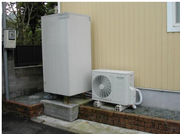
Heating capacity 6kW, tank capacity 460L, 2004 model
