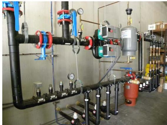
Fig.1 Double pump hydraulic distribution system diagram
