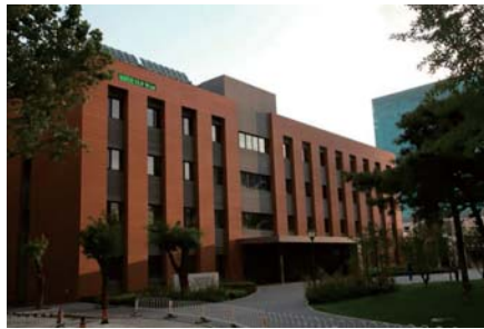
Figure 1 Front view of the nearly zero energy building
