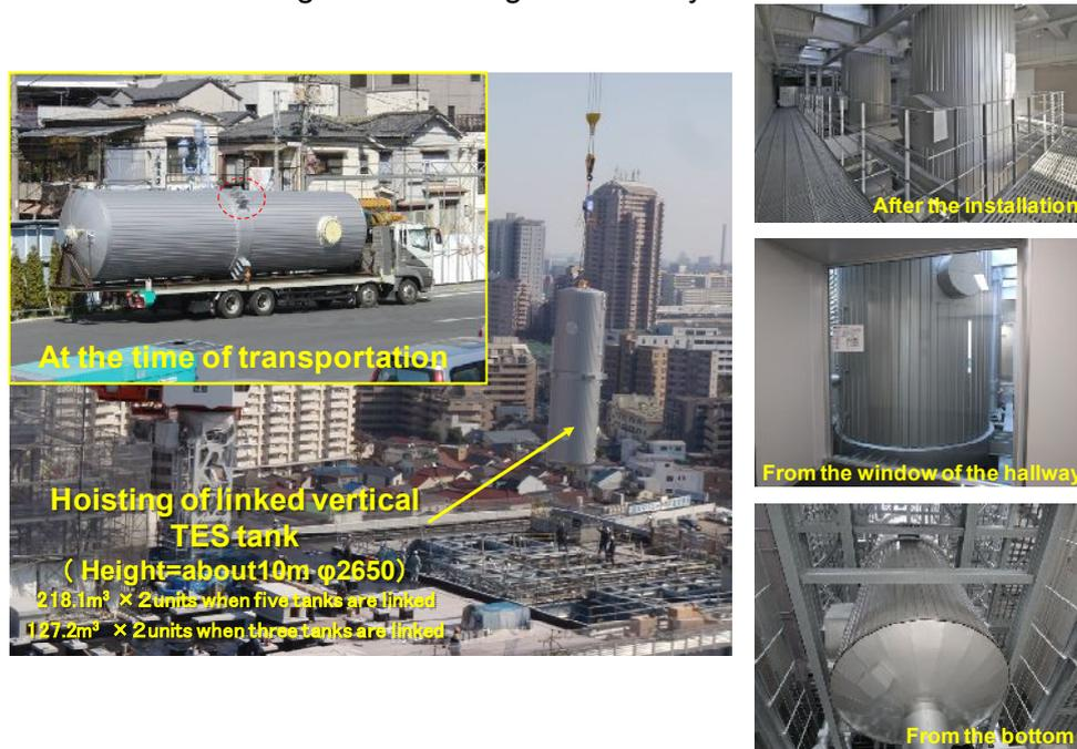
Figure 7: Linked vertical TES tanks
