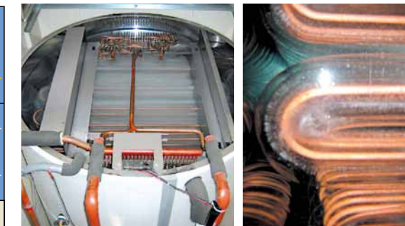
Overall appearance (on the left) and inside (on the right) of ice thermal storage tank
