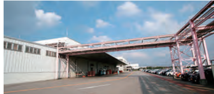
The infrastructure line connecting the first connection building with each facility. With the distance, heat loss was inevitable.
