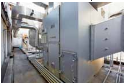
Heat pump unit with VOC processor attached to the upper portion
