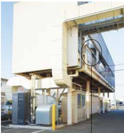
Heat pump unit with VOC processor attached to the upper portion
