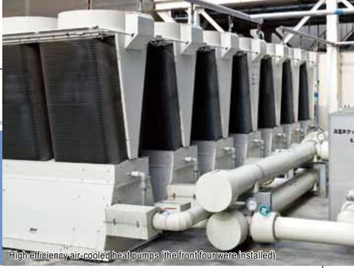
High efficiency air-cooled heat pumps (the front four were installed)
