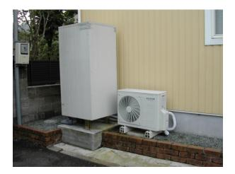
Heating capacity 6kW, tank capacity 460L, 2004 model Fig.8 Eco Cute of my home
