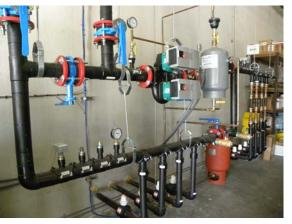
Fig.1 Double pump hydraulic distribution system diagram
